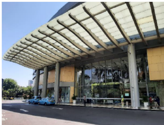
Figure III-3. Sample of Shading Device for Commercial Buildings
