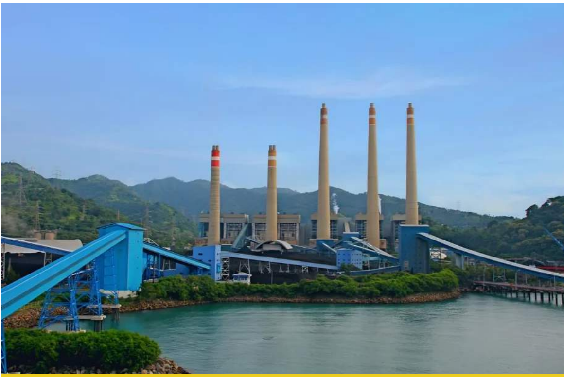
Figure 5-2 Suralaya Power Generation Unit
