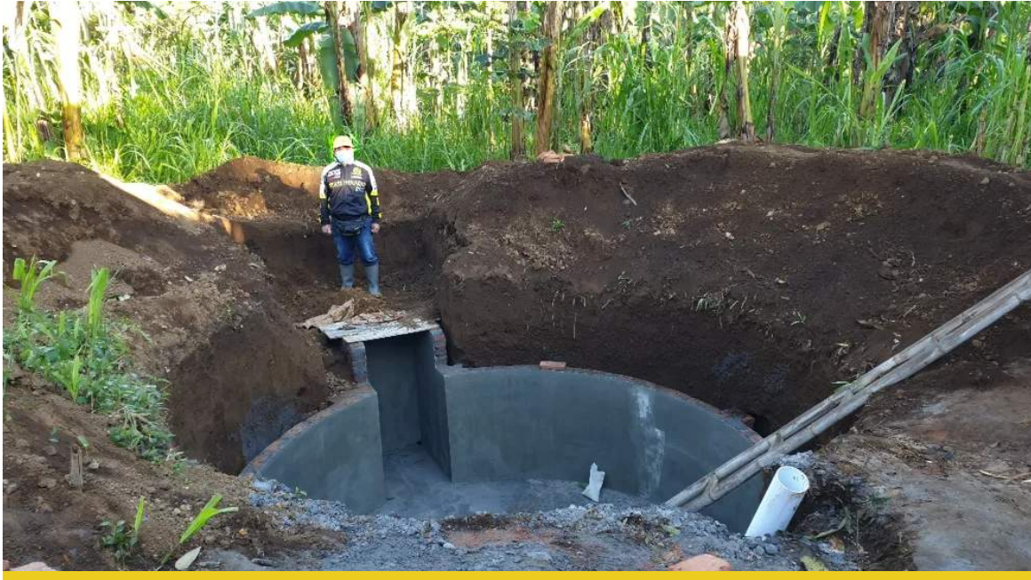
Figure 3-4 Biogas Digester for Households Using Fixed Dome
