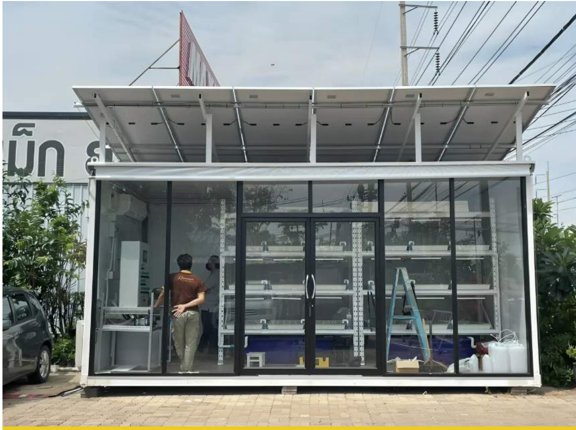
Figure 6-3 Delta's Smart Factory Farm Green House
