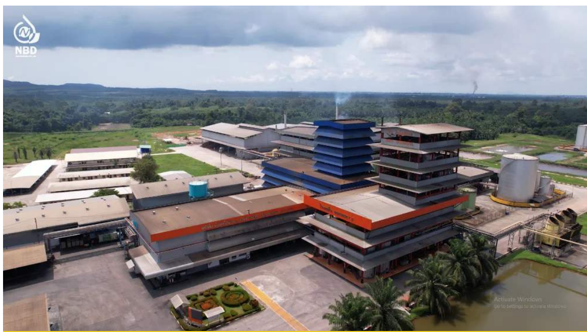
Figure 4-3 New Biodiesel Plant
