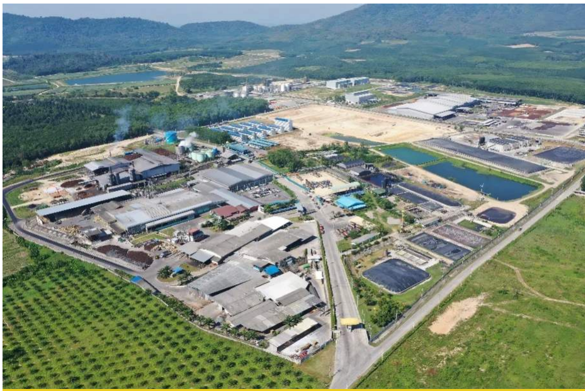
Figure 3-5 Thai Eastern Bio Power Plant
