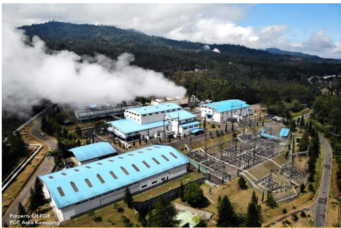
Figure 2-4 Kamojang Unit-5 Geothermal Power Plant
