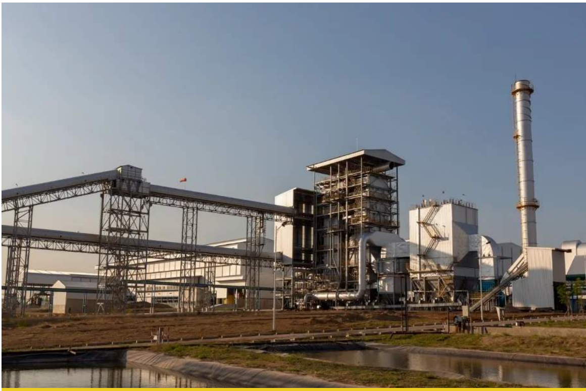
Figure 5-1 ES Energy (Wang Sombun) Bagasse Combined Heat Power Plant
