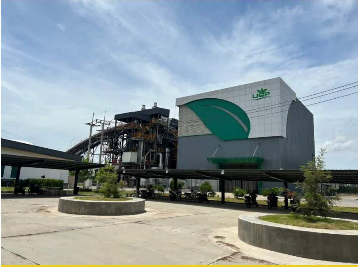
Figure 2-5 Uttaradit Biomass Power Plant
