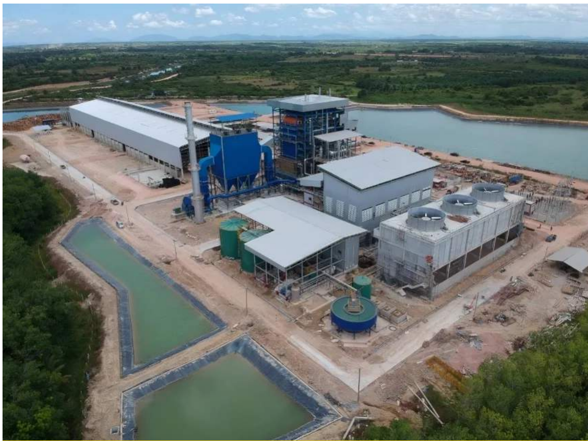
Figure 2-6 Pattani Biomass Power Plant
